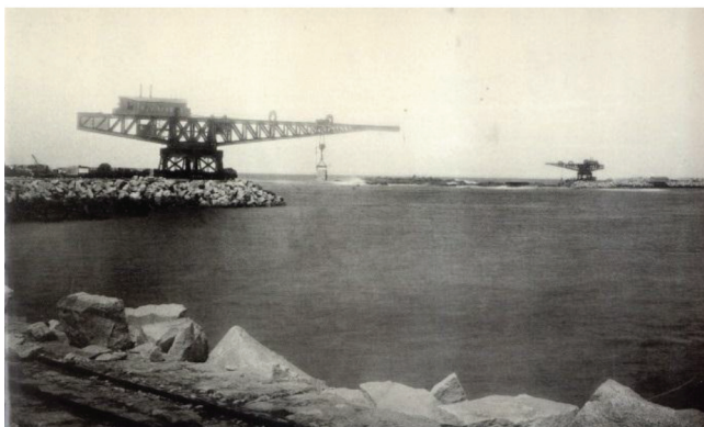
Figure 6: Construction of the Leixões breakwater
