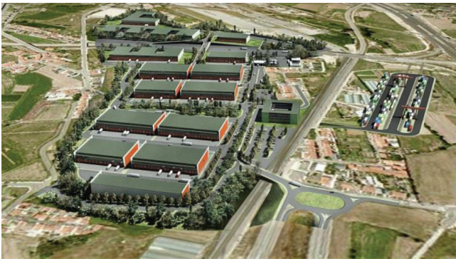
Figure 21: Logistics platform – Site 2
