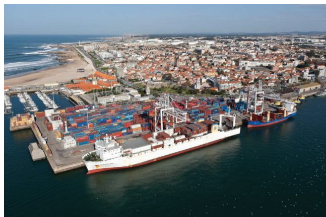
Figure 13: North container terminal
