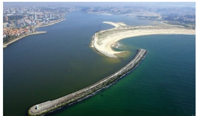
Figure 4: Douro moles at the entrance of Douro River
