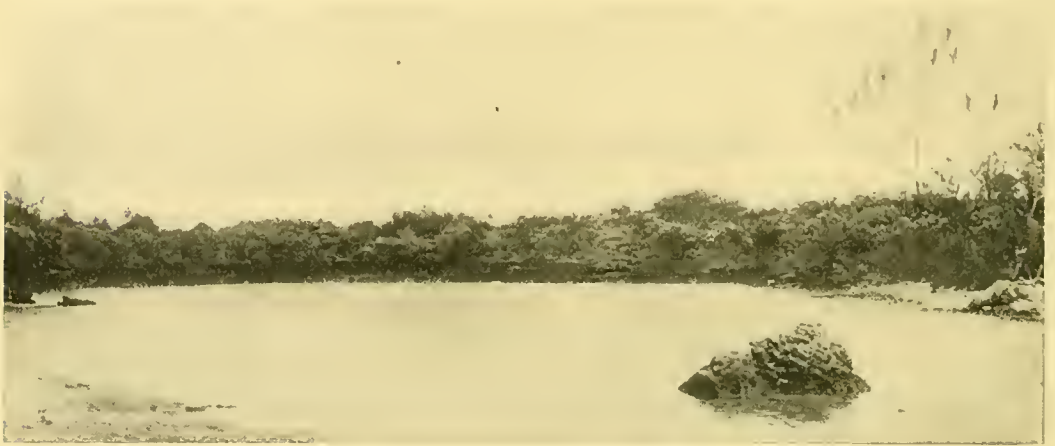
OLD LEDGE DAM AND SPUR, LAGOON SIDE OF WEST COAST OF RANGIROA.
