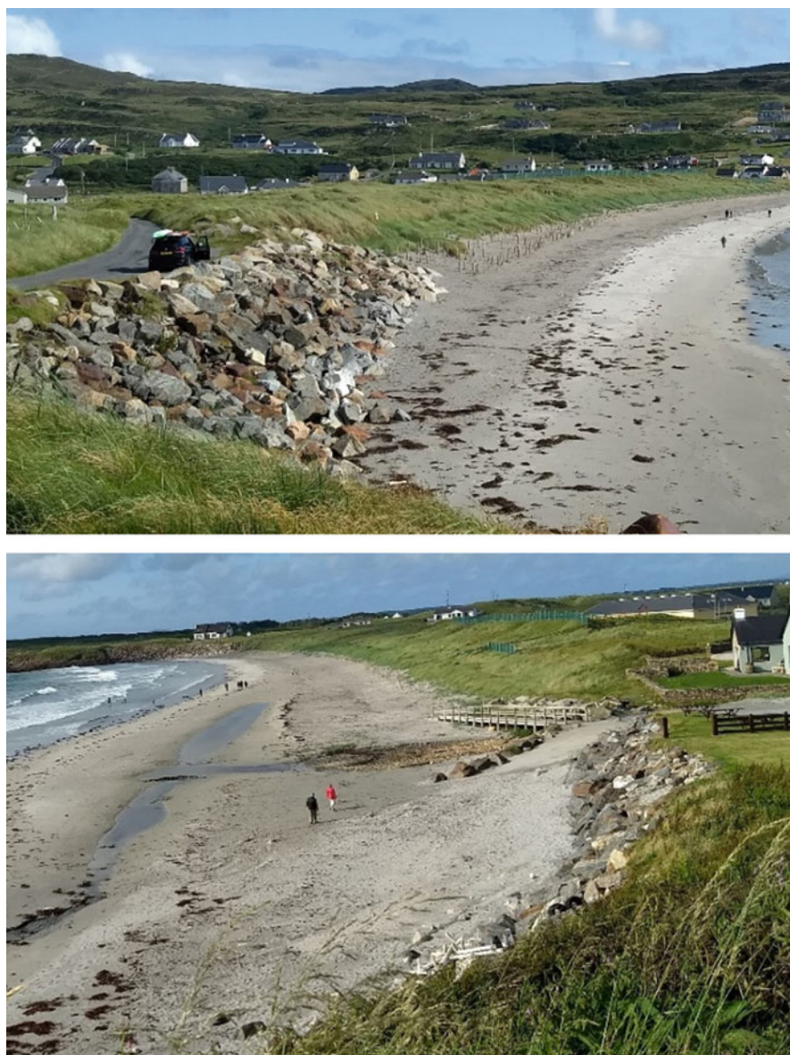
Fig. 32.2 Rock Armour on the northern and southern sides of the beach. (Photo: Paul Lawlor, 2019)
