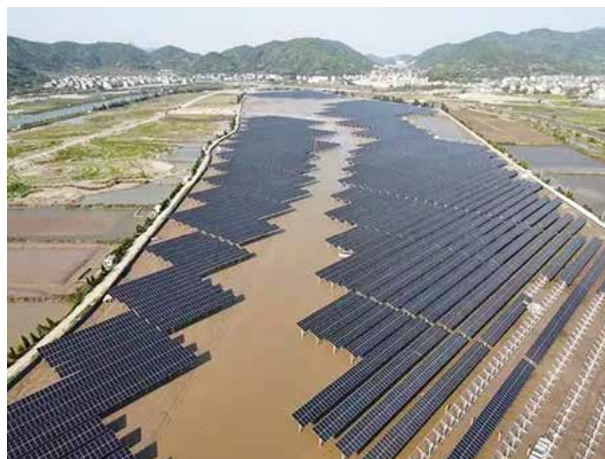
Zhejiang Wenling tidal-PV complementary power station
