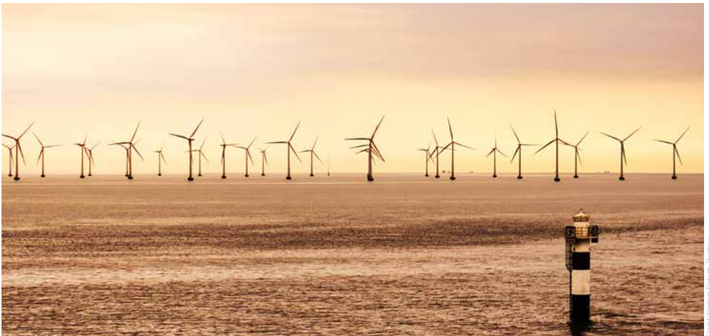
Wind turbines at sea.
