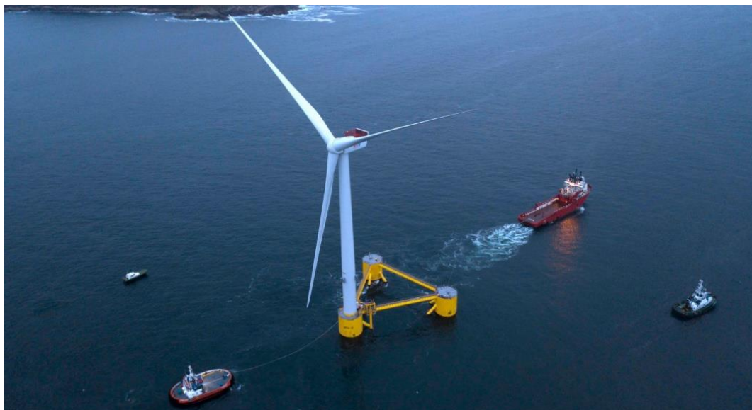
Figure 2.7. Floating turbine being towed for the WindFloat Atlantic project. (Source: WindFloat [19])
