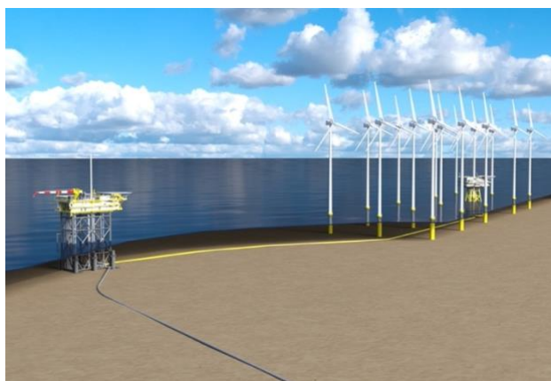
Figure 2. Visualization of the GEMS project showing the N05-A platform location and Riffgat Windfarm including the pipeline and cable route. Retrieved from HSM Offshore Energy (n.d.).
