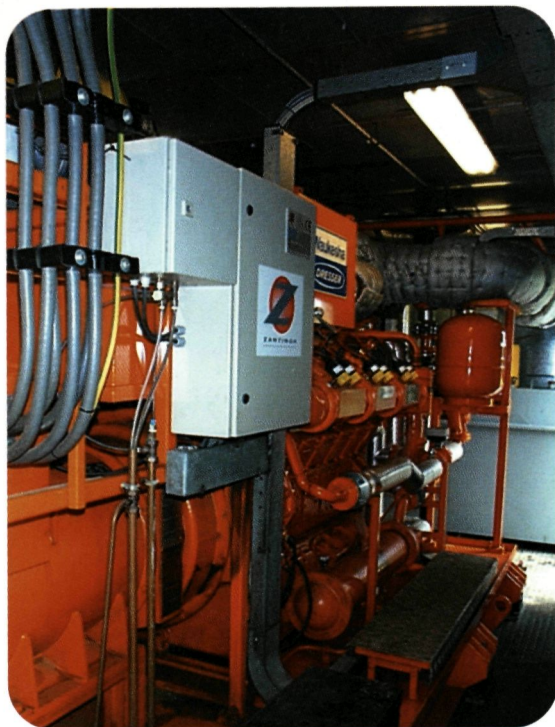
Fig. REG 1: Demonstration of the combined use of heat and power (CHP) in horticulture. The addition of a flue gas catalyst and a condensor allows to use the flue gases for CO 2 fertilisation in the greenhouse.
