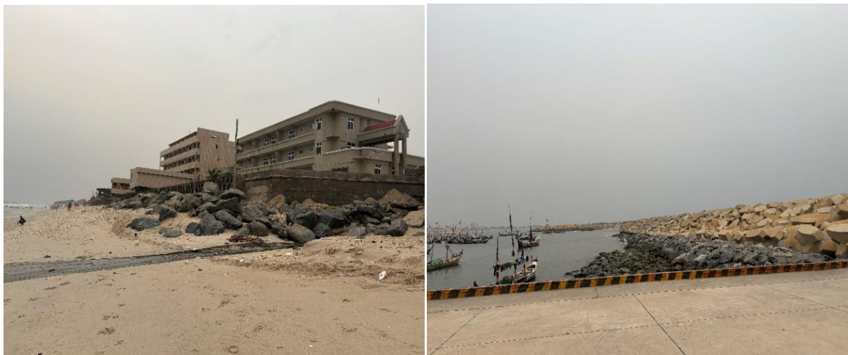
Figure 4.8 Hard Infrastructure (seawall and groins) constructed at JamesTown and Teshie
