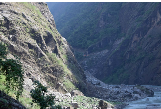
Fig. 71 Typical rockslide observed at Upper Tamakoshi Hydropower Station triggered by the Gorkha Earthquake
