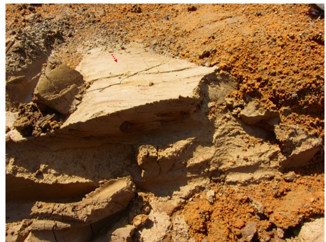
Fig. 22 Slickensides observed in the slid mass at Hanokidaira Landslide
