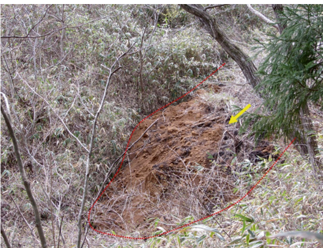
Fig. 28 Toe of Yamabe Landslide
