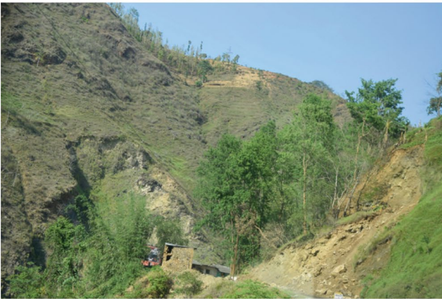
Fig. 55 Typical failure along Araniko Highway due to river undercutting and earthquake shaking
