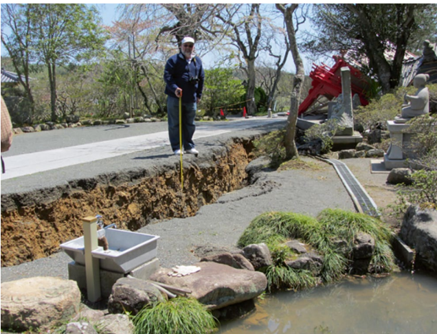
Fig. 3 Fault rupture at Kantokuji Shrine
