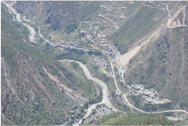
Fig. 83 Landslide mass blocking roads and threatening to block stream flow
