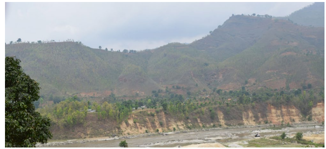
Fig. 51 Landslides along river bank opposite from Prithivi Highway
