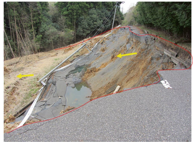
Fig. 16 Landslide in the Sorihata area
