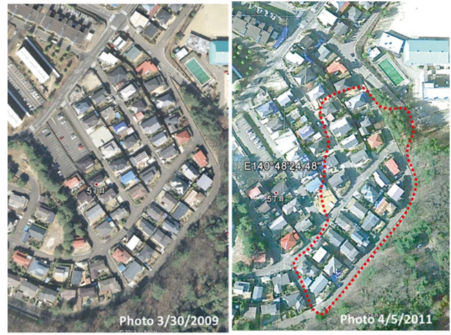
Fig. 33 Google Earth images of the Oritate Residential Area prior to and after the earthquake (locations a and b are the locations of photographs in Figs. 34 and 35)
