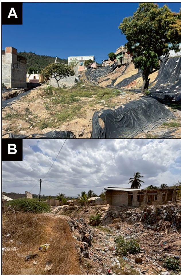
Fig. 1 Landslide disaster risks are created at the nexus of human livelihood activities. (A) is the case of a risky slope in Tegucigalpa, Honduras, where many houses have been erected; (B) is the gully erosion, which has been active due to uncontrolled house constructions in Nacala city, Mozambique. (Photos were taken by the author)
