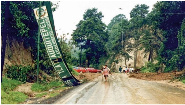
Fig. 2 Damage following the rainfall events of October 1999 https://laruleta.com.mx/la-tragedia-que-marco-a-los-serranos/
