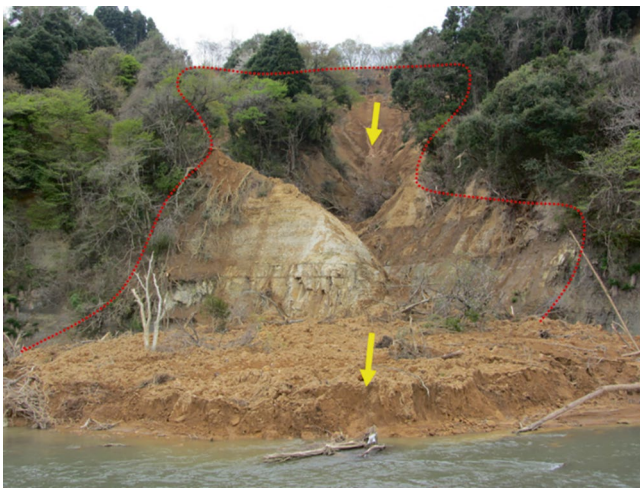
Fig. 39 Photograph of the Arakawa Landslide taken after the earthquake
