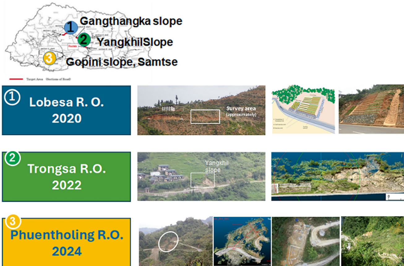
Fig. 5 Three Bioengineering sites in Bhutan
