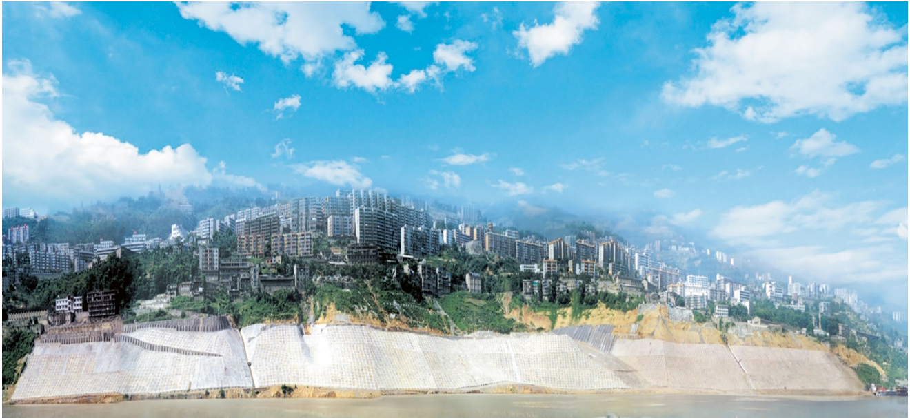
Fig. A.12 Photo of old Badong County, showing the populated area built on the Huangtupo landslide (Tang et al. 2015a)
