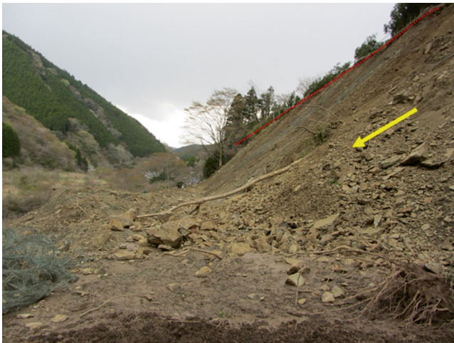
Fig. 11 Damage at the Saibachi Rock fall
