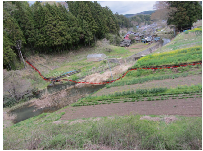
Fig. 4 Ground rupture near Tabito Junior High School, Location b in Fig. 2
