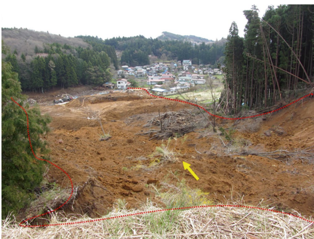
Fig. 20 View of Hanokidaira Landslide from top
