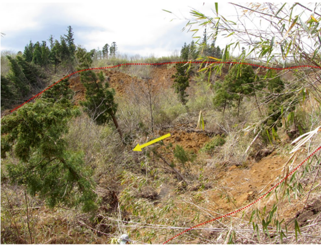
Fig. 26 View of Yamabe Landslide from top
