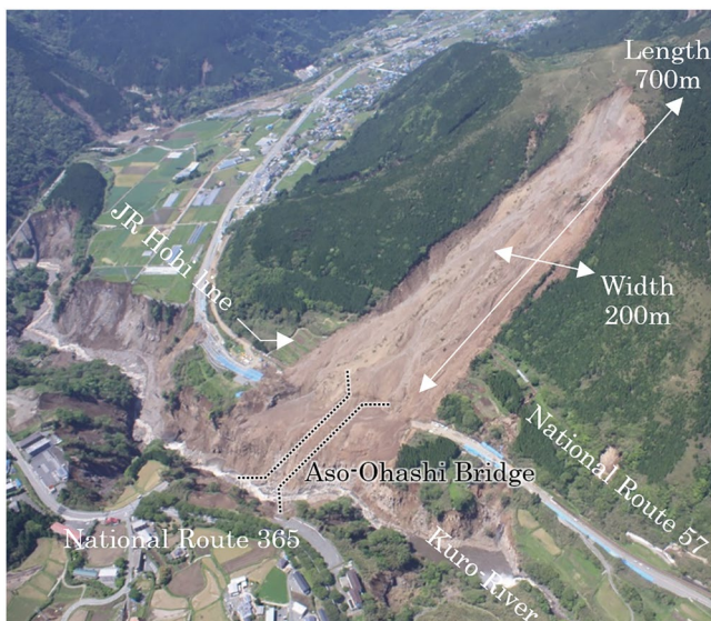
Fig. 25 A slope failure induced by the mainshock near the Aso-Ohashi Bridge (Modified from the Kyushu Regional Development Bureau, MLIT 2021). (Fig. 10 in Higaki et al. 2023)
