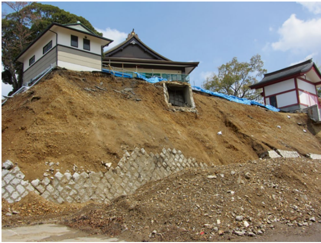
Fig. 47 Damage of retaining wall of a shrine observed in Mito City
