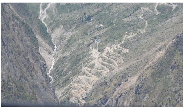
Fig. 85 A portion of the river blocked by landslide debris
