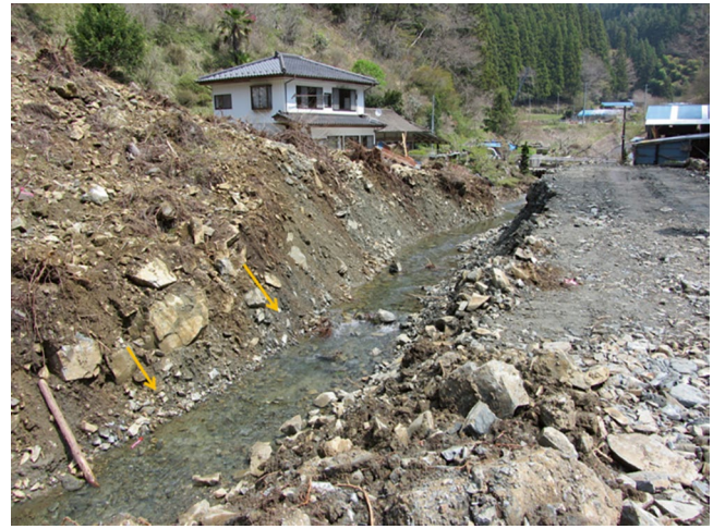
Fig. 37 Stream that was blocked by Kaiya Landslide
