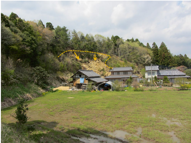
Fig. 43 Rock slide that damaged three buildings in the Naka area
