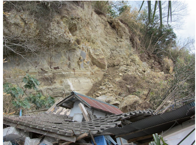
Fig. 46 Typical rockfall observed in Matsushima Island
