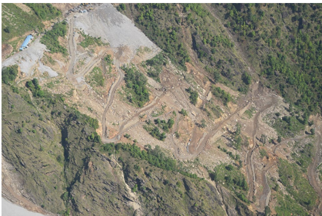
Fig. 63 Typical landslides triggered by the 2015 Gorkha Earthquake along the rural road alignments
