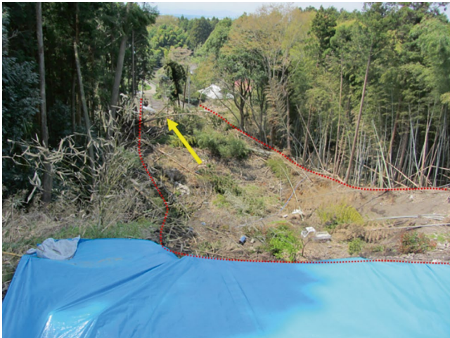
Fig. 32 Landslide damage at location ID 2 in the Kashiwazaki Residential Area
