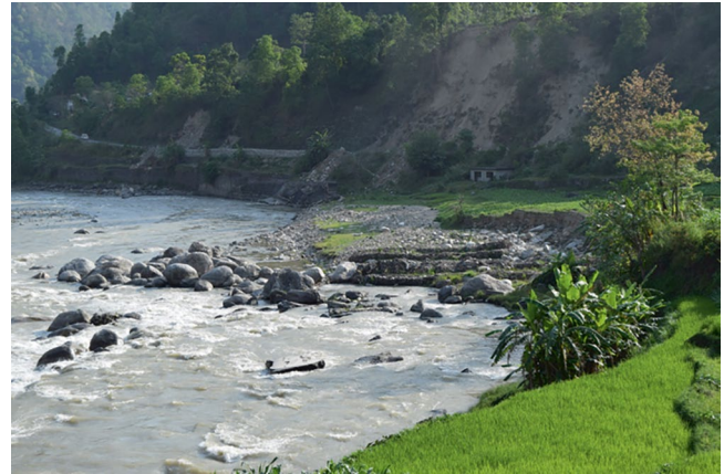
Fig. 55 Typical failure along Araniko Highway due to river undercutting and earthquake shaking
