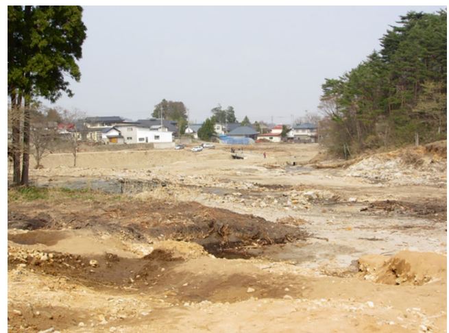
Fig. 50 Damage sustained at the downstream due to the collapse of Fujinuma Dam
