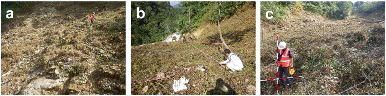
Fig. 14 Measuring at Gopini slope on January 3, 2024 ((a) upper part of the site, (b) measuring the cascade drain dimension, (c) measuring the ground height)
