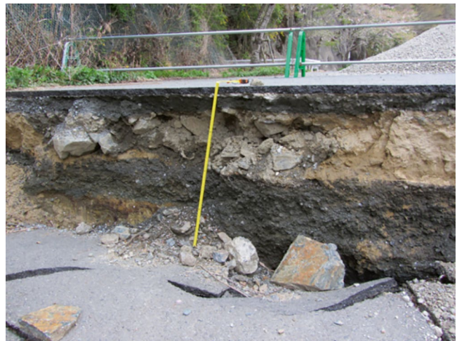
Fig. 5 Photograph at the location a, Gosaisho Highway in Fig. 2
