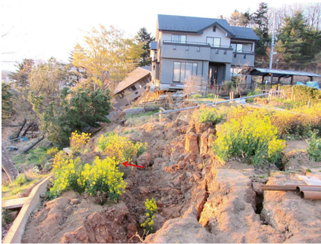
Fig. 36 Collapse of buildings constructed on fills near Sendai City
