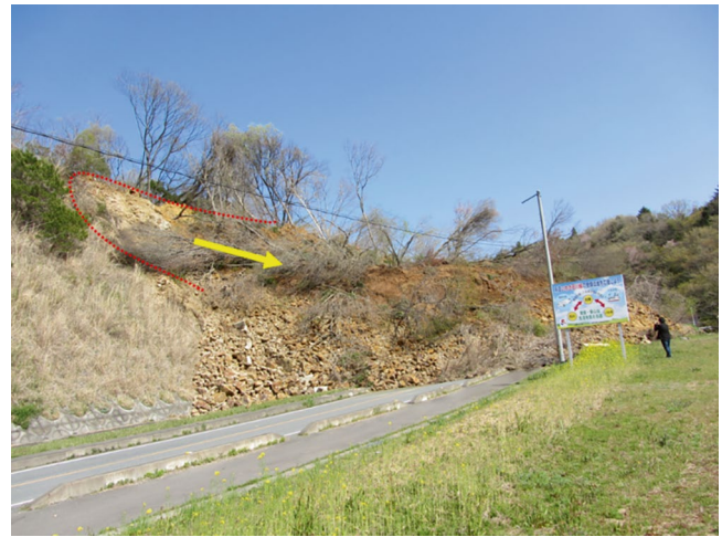
Fig. 29 Overall view of Watanabe Landslide
