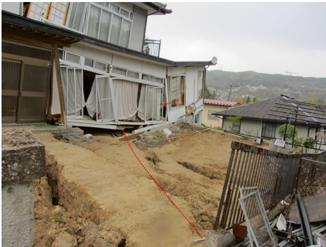
Fig. 35 Collapsed building in Oritate Residential Area (location b)
