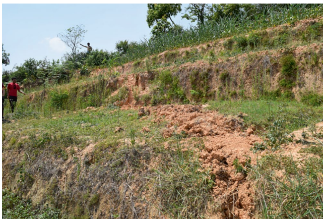
Fig. 73 A long crack observed along the mountain ridge at Ramkot Village near Kathmandu
