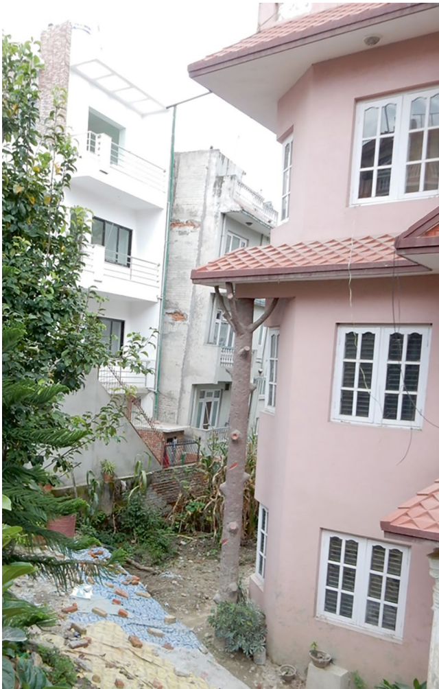
Fig. 91 Tilted buildings along the main scarp of the Lokanthali ground failure site
