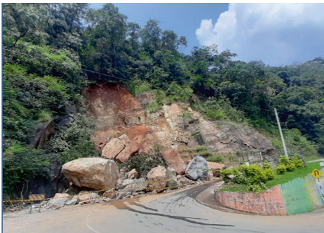
Fig. 4 Rock falls in Kandy–Mahiyangana Road (Credit NBRO)
