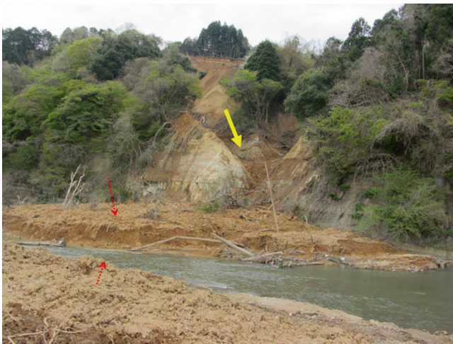
Fig. 40 Landslide dam formed at the Arakawa Landslide after the earthquake
