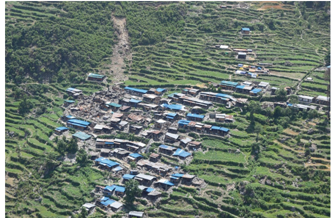
Fig. 66 Typical landslides triggered by the 2015 Gorkha Earthquake along the Dhunchhe Road that was threatening the community
