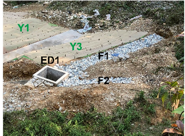
Fig. 17 A French drainage F1 (l = 9.1 m), F2 (l = 4.0 m) (left: cross-section: right: Bird's-Eye view of the French drains) drain)
