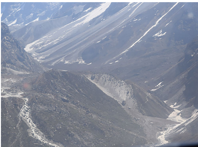
Fig. 84 River blocked by the landslide debris
