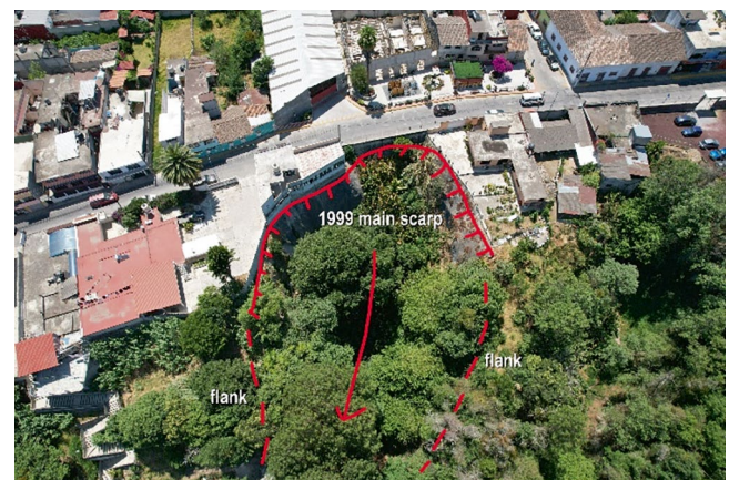
Fig. 12 Homes with shotcrete walls, 2023. Drawn lines indicate the main scarp and flanks of the past landslide. (Photo courtesy of Ricardo J. Garnica-Peña)
