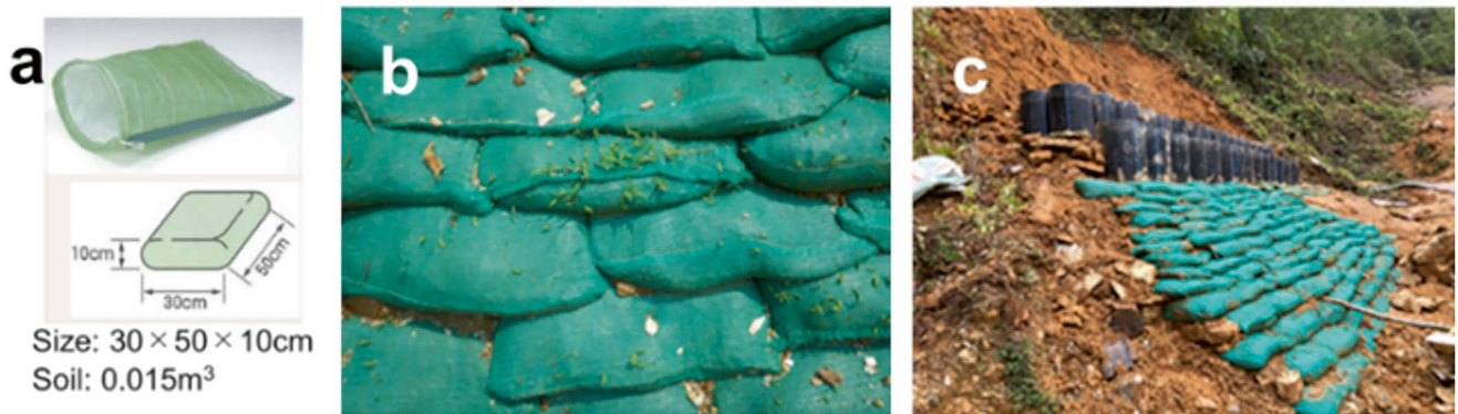
Fig. 43 Sandbag planting ((a) materials, (b) piled seeds bags, (c) sandbag layout)
