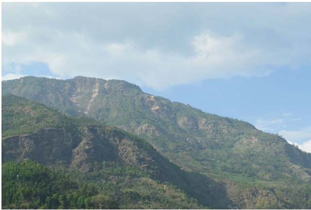
Fig. 58 Landslides along the top of the ridge that are threatening Araniko Highway and Sunkoshi River
