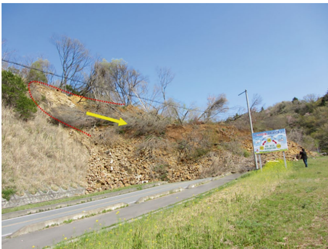
Fig. 8 Watanabe Landslide located near the Yunodate fault rupture area
