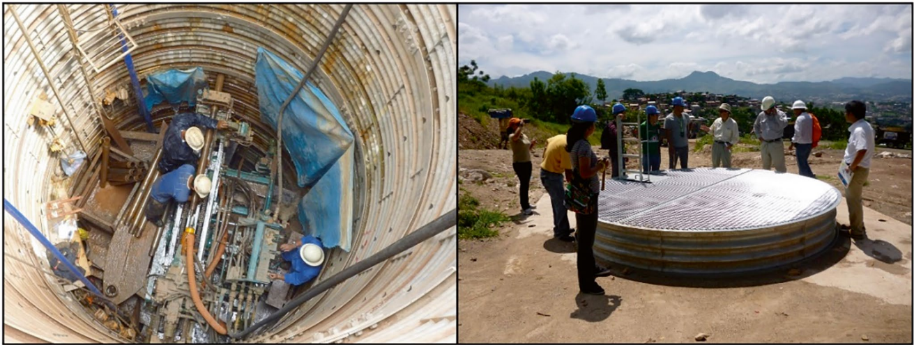
Fig. 5 These are photos of the water catchment wells installed in El Berinche, under the grant aid project. Even now, the wells function appropriately while keeping the safety factor at a safe level. (Taken by Hirota, K.)
