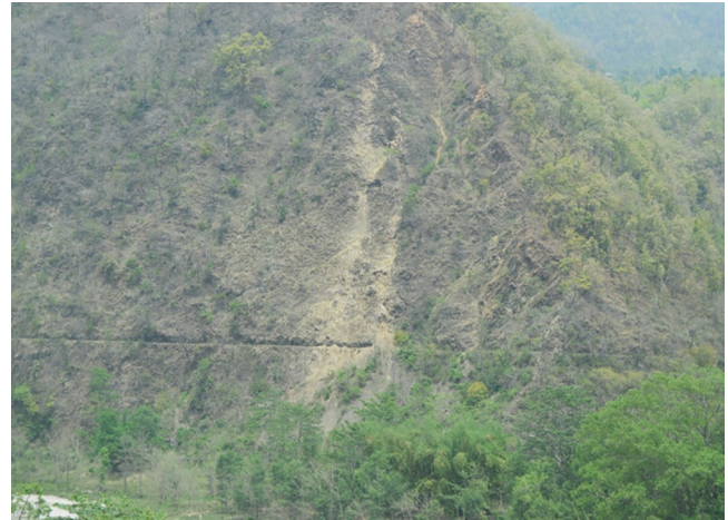
Fig. 52 Landslide along an irrigation channel located opposite to the Prithivi Highway
