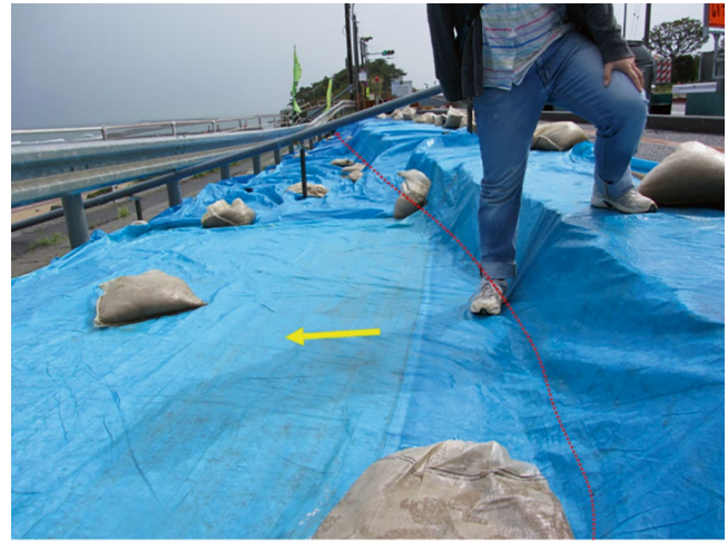
Fig. 45 Coastal landslide observed near Hitachi Bay
