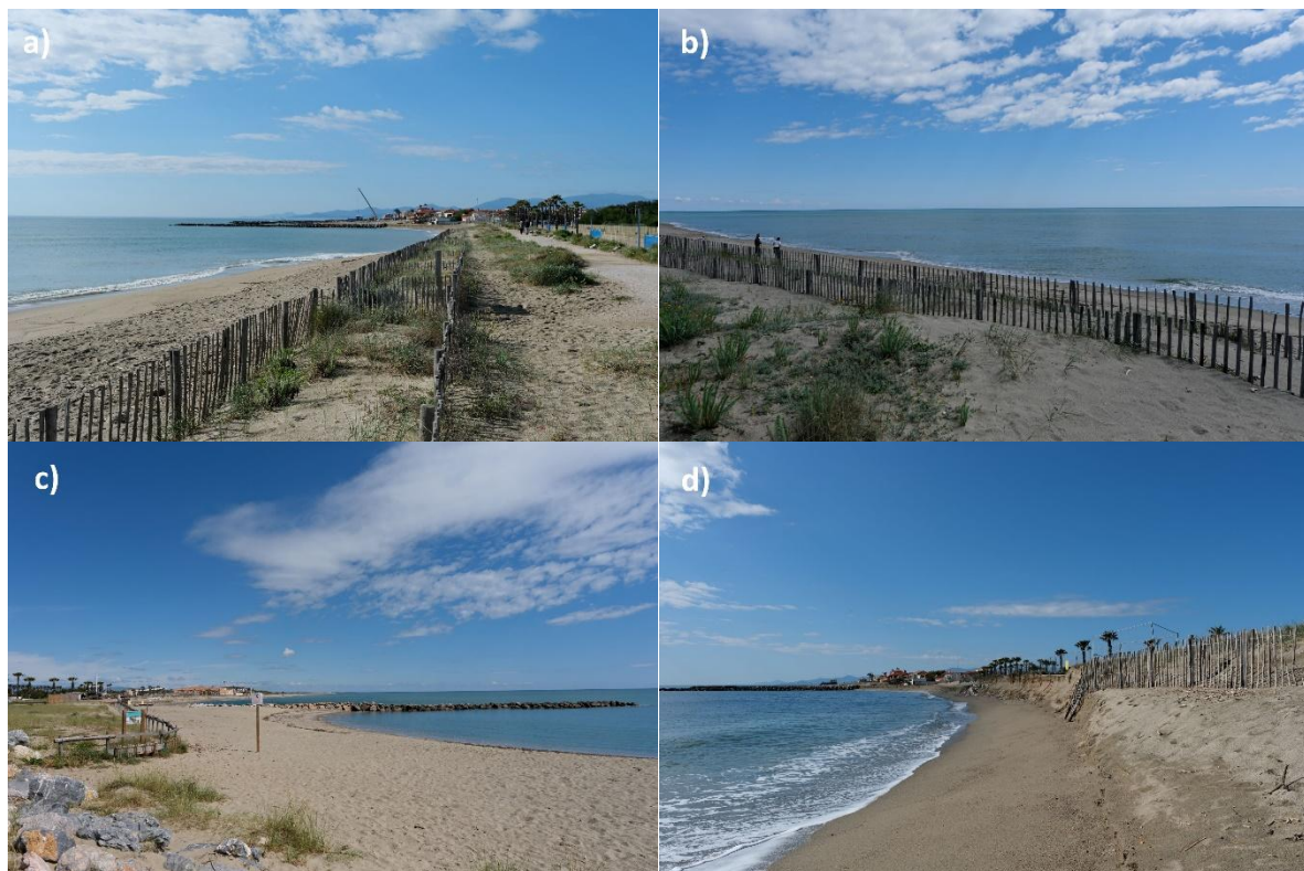
Figure 12 Sainte-Marie-La-Mer (FR) demonstrator – a) sand fences with naturally established vegetation; b) sand fences from another angle; c) groin extending into the sea near the demonstrator; d) severe erosion with fences having fallen into the sea.
