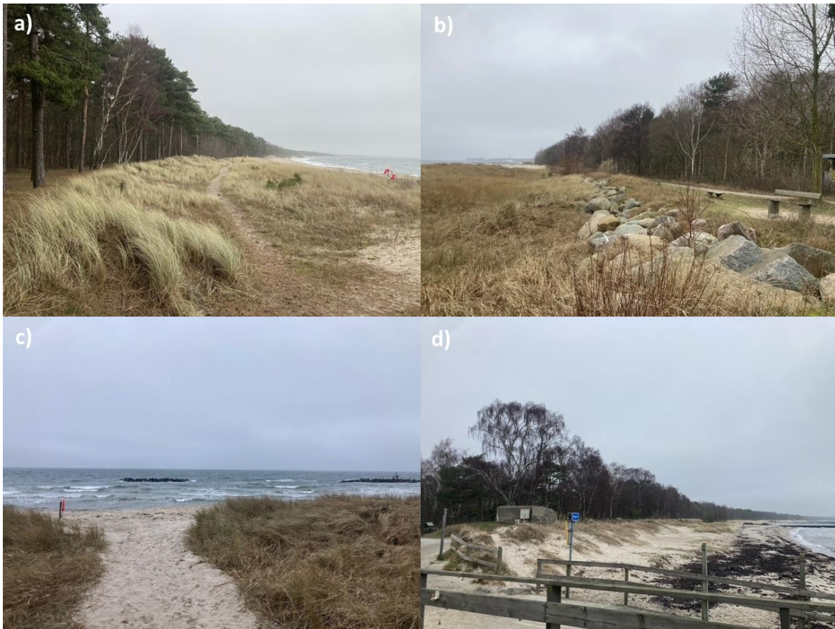
Figure 2 Ystad (SE) demonstrator: a) dune landscape in front of a conifer forest; b) rock revetment gradually being covered by dunes; c) path between dunes leading to the beach; d) beach viewed from a small dock.
