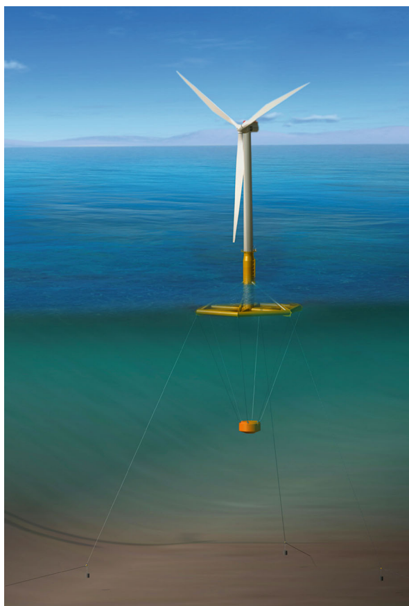
Fig. 3 A schematic view of Hexafloat turbine and its mooring system
