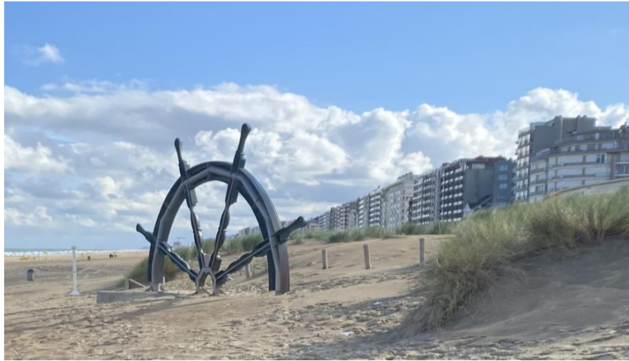
Figure 2. Example of Dune-Dike hybrid Nature-based-Solutions at Westende, Belgian Coast ( Stratigaki et al., 2024 )
