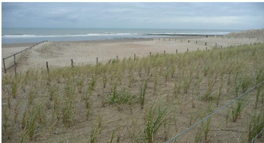
Figure 1. Marram grass Dune-Dike at Westende, Belgian Coast (Stratigaki et al., 2024; photo courtesy Herman Troch)
