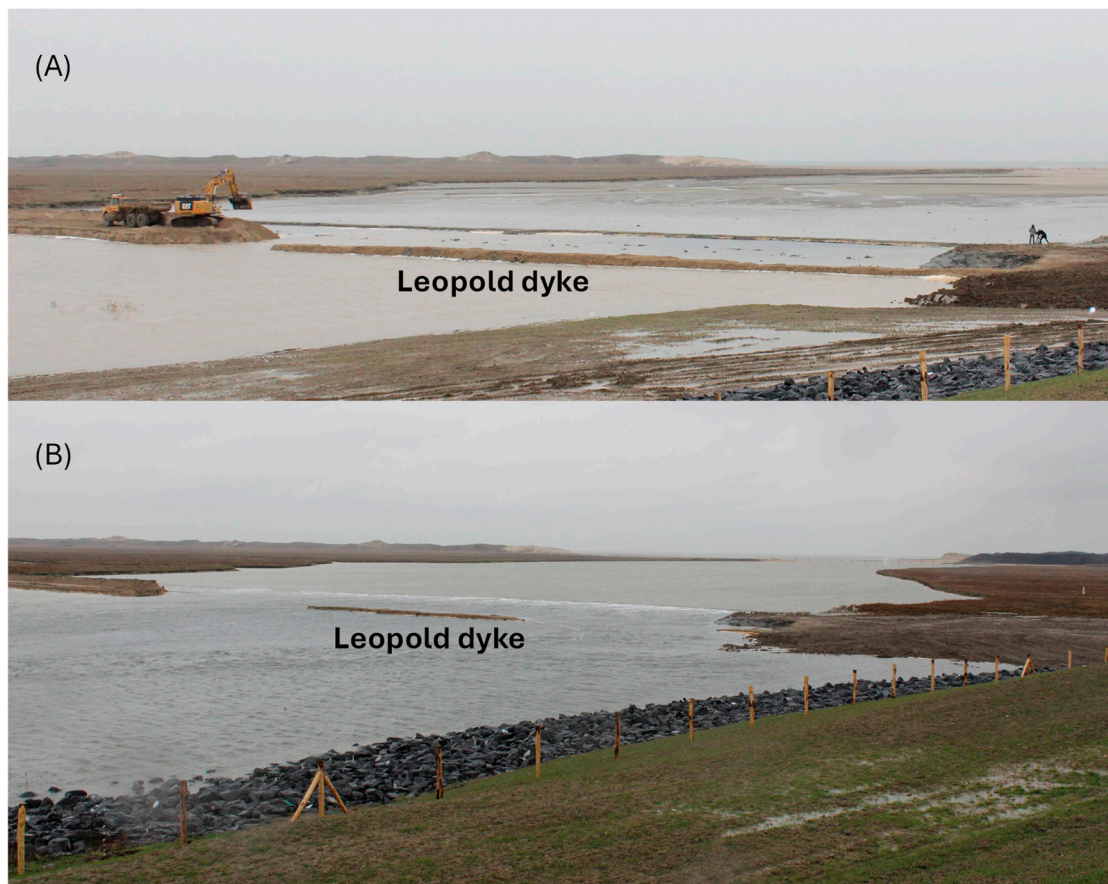
Figure 2. Opening of the dyke on 4 February 2019. (A) During the beaching of the dyke; and (B) few hours later. Figure 1 displays the location.
