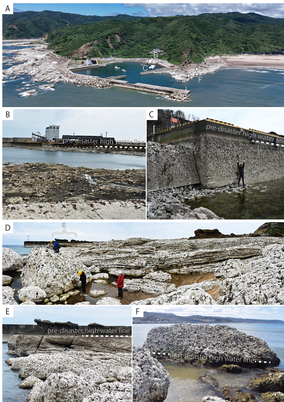
Fig. 1. A: The landscape around Kaisei fishing port (B, C) and our main study site, Kaisei Reef (D–F). (B) Exposed sea bottom surface due to uplift; (C) The uplifted harbor wall; (D) Kaisei Reef whose surface was covered with whitened algae remains. Note that the current sea surface was at the feet of the authors. (E) The presumed pre-disaster coastline coincides with the horizontal line between the blackish and whitish areas. (F) Green algae covering the current coastline. A was photographed on July 11, 2024. B, D, and E were taken on April 21, 2024. C was on March 21 and F was on March 27, 2024.
