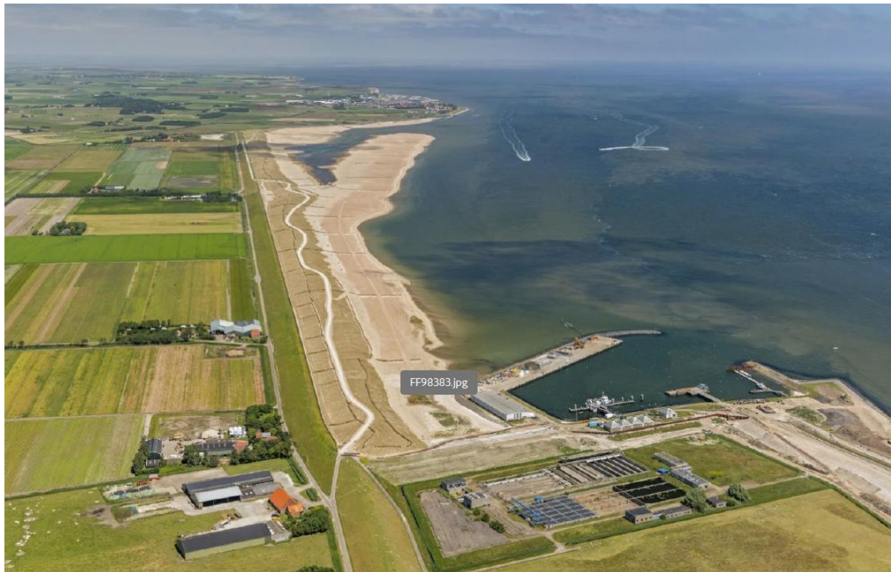
Figure 5: Texel, Prins Hendrik Zanddijk (NL) Demonstrator, Dune-in-front-of-Dike
