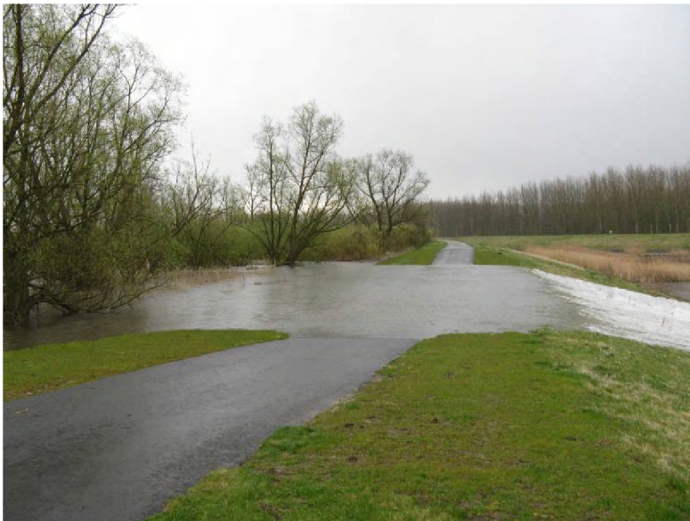
Photo 1. Lowered overflow dike of Lippenbroek in action.
