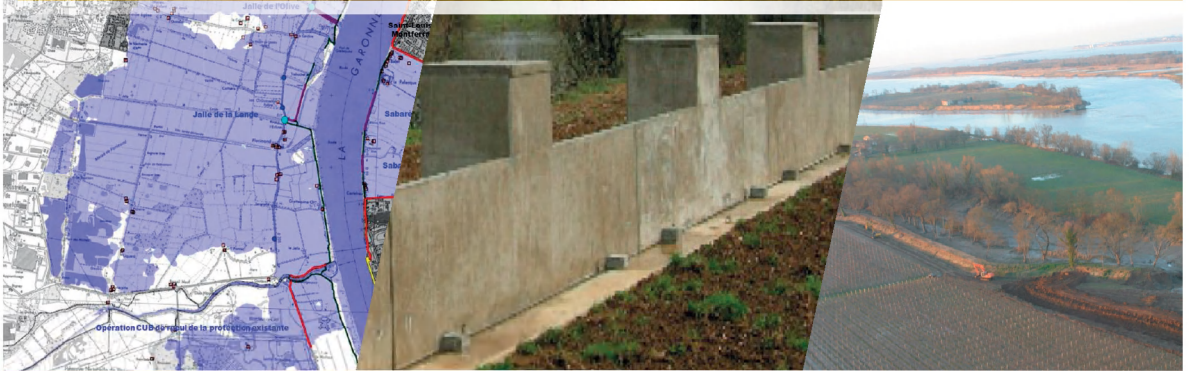
Illustration of the existing protection for identified problem areas: Blanquefort Marsh
