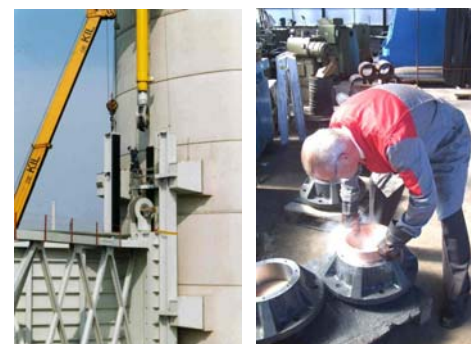
Fig. 2. UHMPE guides of the Hartel Canal Barrier and Tenmat® pivot bushings of the Naviduct miter gates, Enkhuizen
