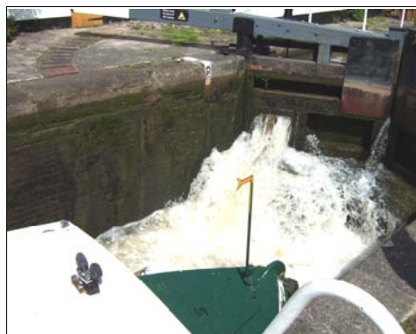
Figure 1: Through-the-gate filling on a canal near Chester / Great Britain
