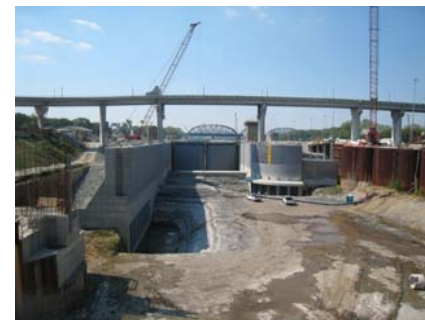
Fig 1: Intakes at new McAlpine Lock during construction
