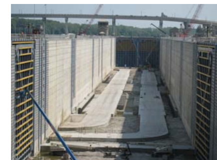
Fig 2: In-chamber longitudinal culverts, McAlpine Lock
