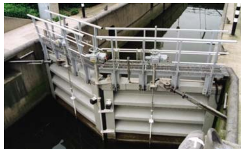
Fig. 1. FRP gate of a lock near Werkendam
