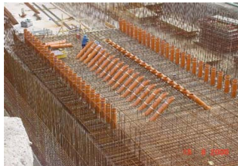
Picture 1: Permanent formwork for the pressure chamber of Sülfeld lock
