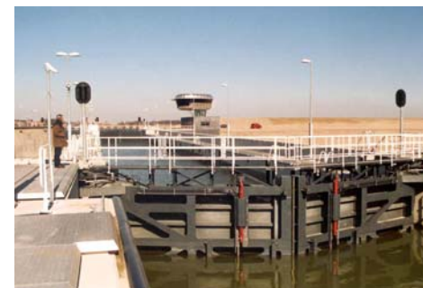
Fig. 2. Miter gates of the Naviduct in Enkhuizen, carrying reverse water head
