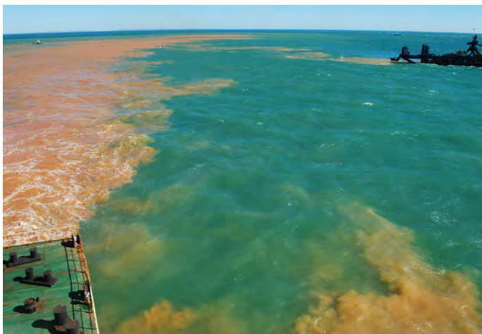
Figure 1. Dredging plume releasing turbid water in clear ambient waters. (Photo: courtesy of EcoShape)
