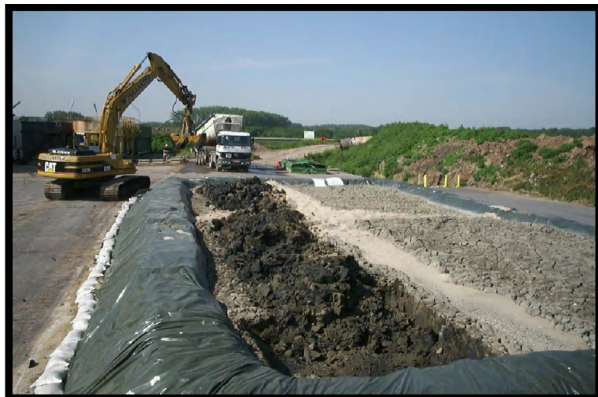
Lagooning of sediments: test field
