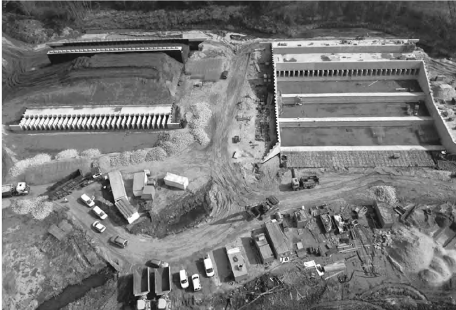
Fig. 8. Aerial view of an actual CRT construction along the Schelde estuary. Photograph shows outlet (left) and inlet (right) construction which will allow implementation of CRT on several hundreds of hectares of lower agricultural land.
