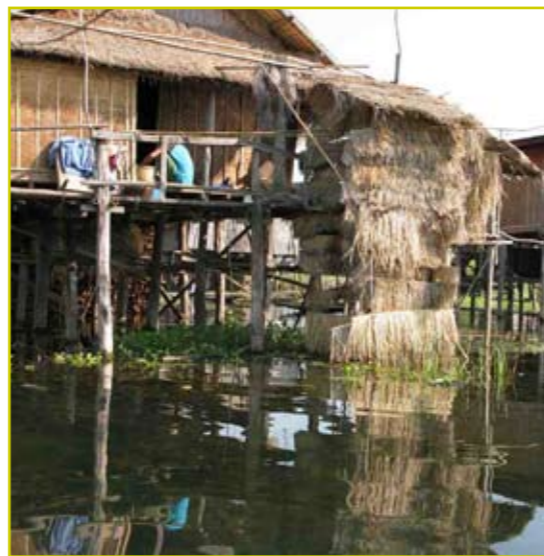
Figure 7.8. A 'flood proof' house constructed on poles in Indonesia.
