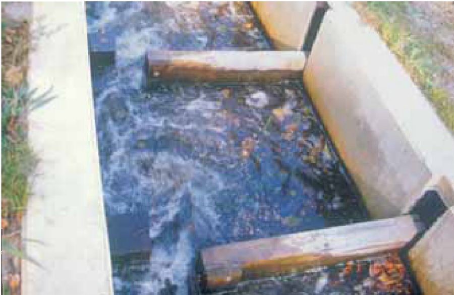
Figure 5.20: Slot current in a slot pass
