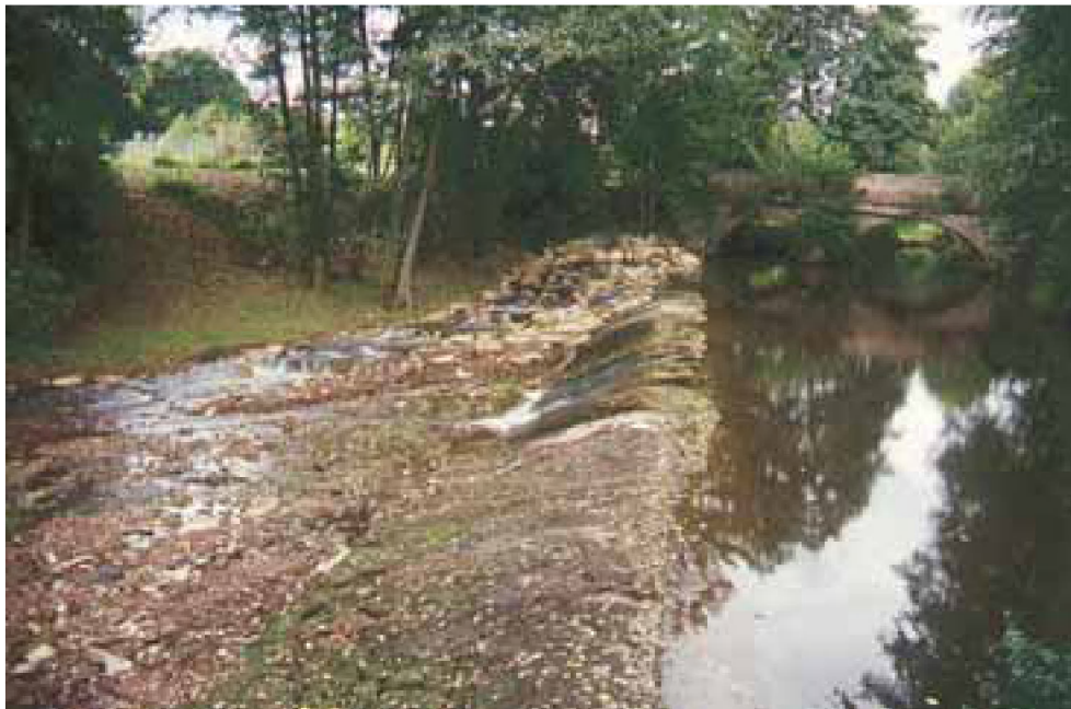
Figure 4.33: Eselsbrücke fish ramp on the Elz (view from tailwater)
