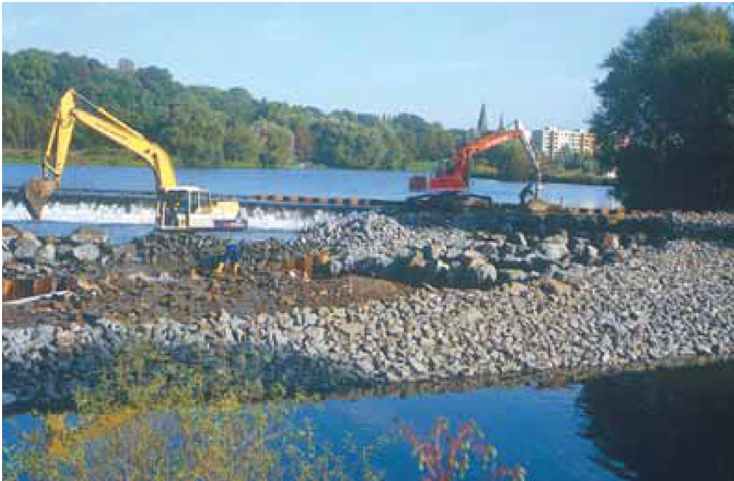
Figure 4.40: Spillenburg weir; fish ramp under construction
