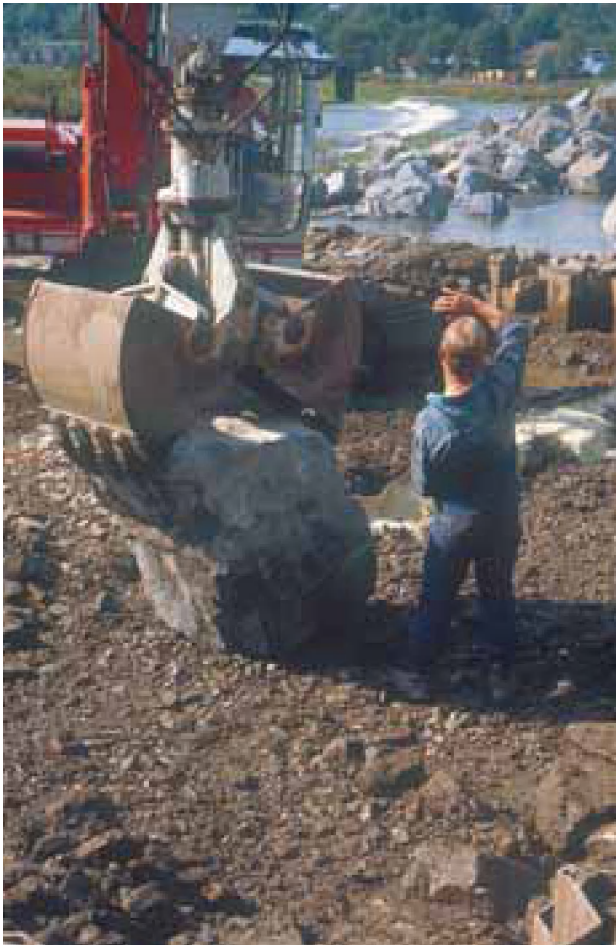
Figure 4.38: Setting the boulder bars
