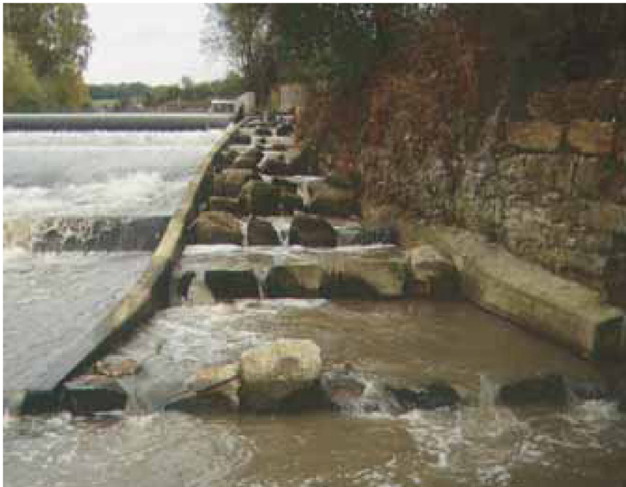
Figure 4.37: Uhingen/Fils rough-channel pool pass View from tailwater end.
