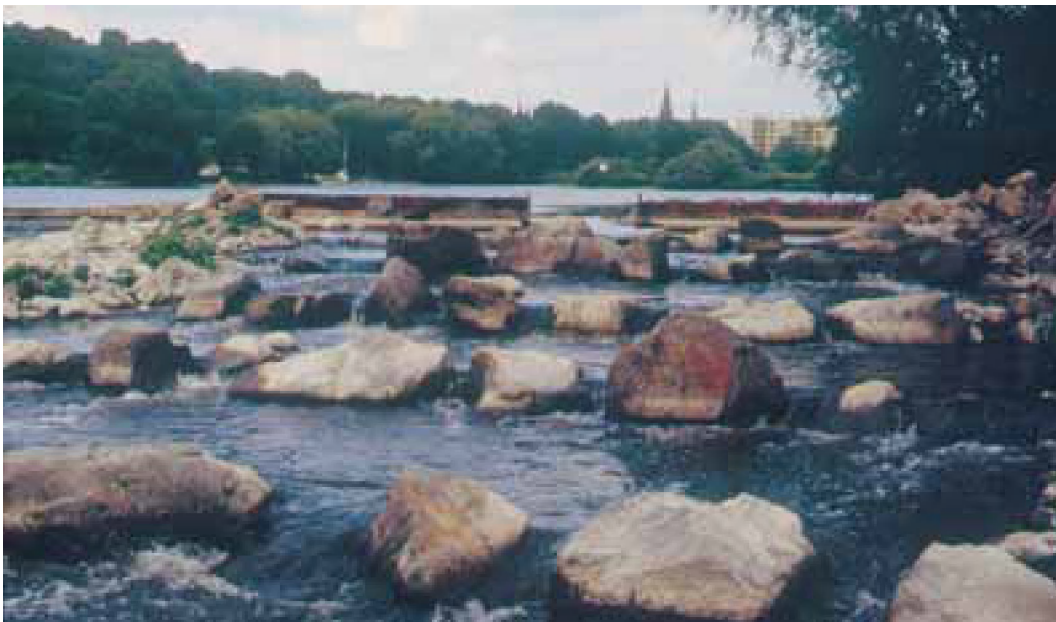
Figure 4.41: Spillenburg weir; fish ramp after completion
