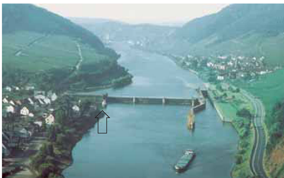
Figure 3.3 Aerial view of the Neef dam in the Moselle River (Rhineland-Palatinate) to show the size of the fish pass (see white arrow) in comparison to the total size of the dam.
