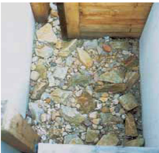
Fig. 3.14: Coarse bottom substrate in a slot pass; Lower Puhlstrom weir in the Unterspreewald (Brandenburg)
