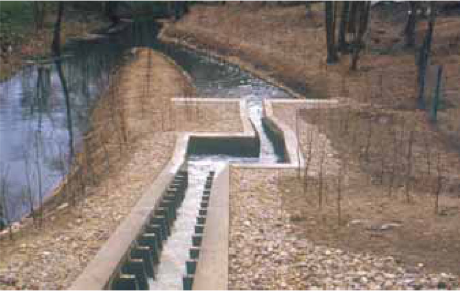
Figure 5.29: Denil pass with intermediate resting pools. View from headwater, Gollmitzer mill/Strom at Prenzlau (Brandenburg)
