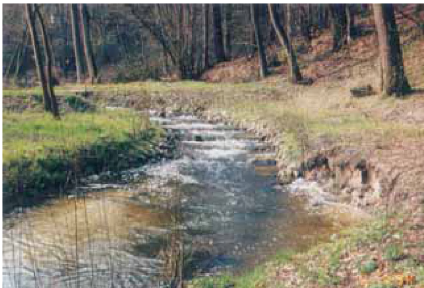
Figure 4.24: Bypass channel at Seifert's Mill
