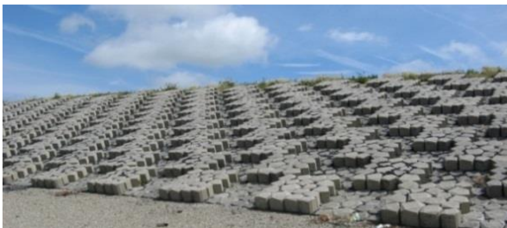
Figuur 1.1: Basalton steenzetting in dambord patroon met ongeveer 20% overlap
